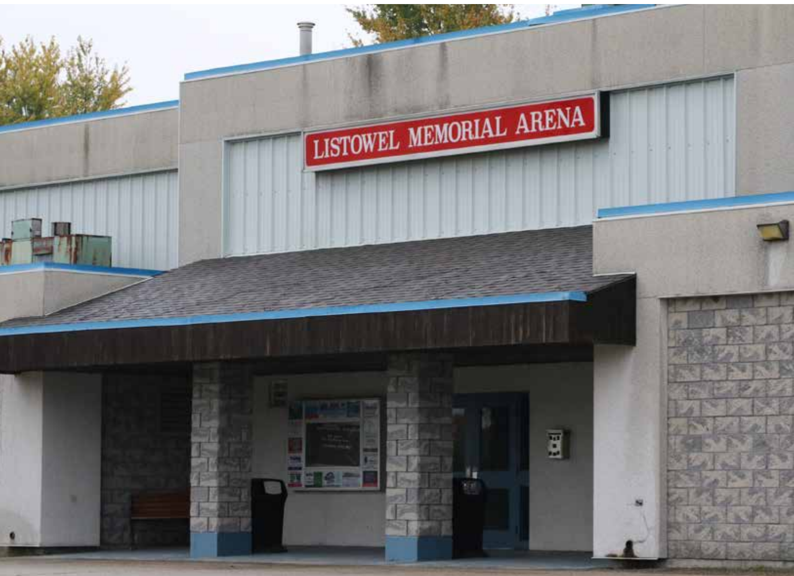
The municipality has announced plans to demolish Listowel Memorial Arena. Photo by Ben Forrest
